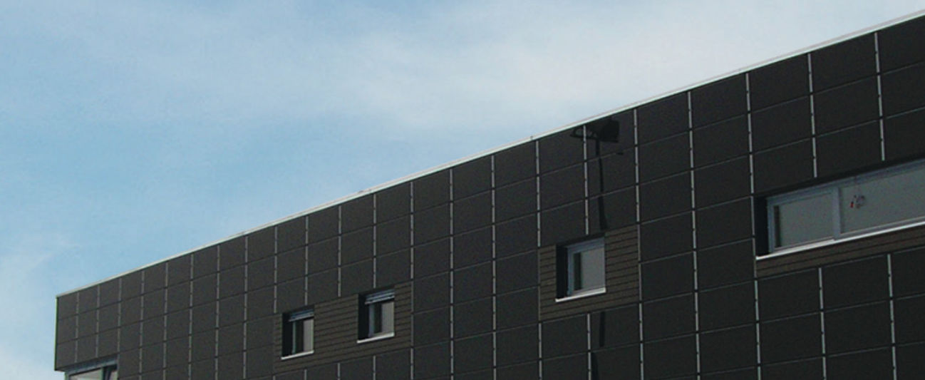
Using facade surfaces optimally
