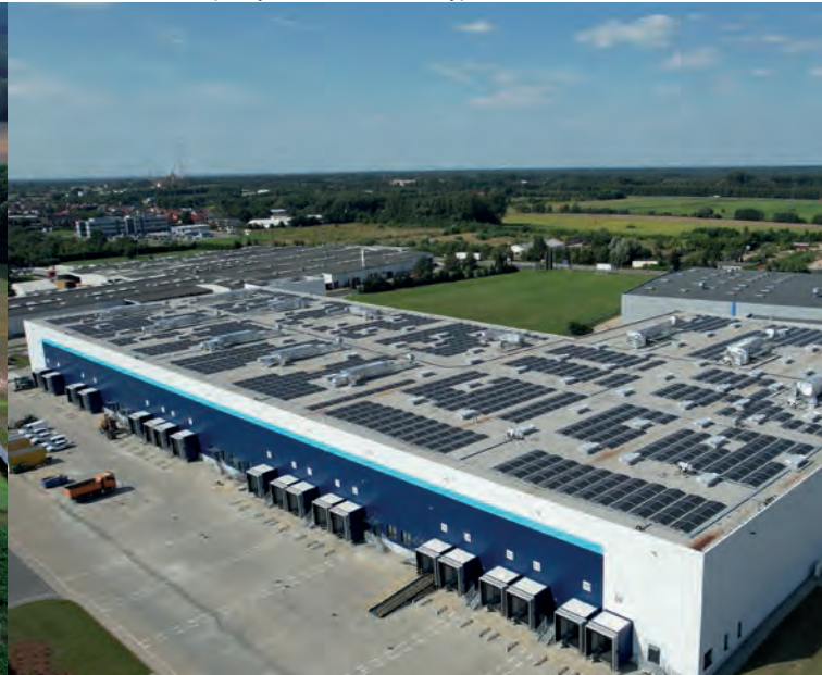
MSZCZONÓW, capacity 1MW, structure type: DP-DNHBE- WZ- 10°
