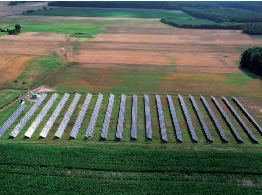
BASZYN, capacity 1MW, structure type: W-H4G2-BI
