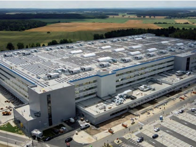
ŚWIEBODZIN, capacity 1,8 MW , structure type: DP-DNHBE- 15°, DP-DNHWE - 15°
